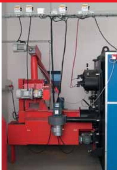
Feeding of wood pellets into the stoker
